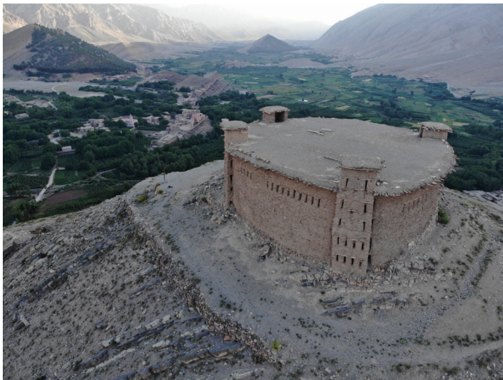
Sidi Moussa granary attic
