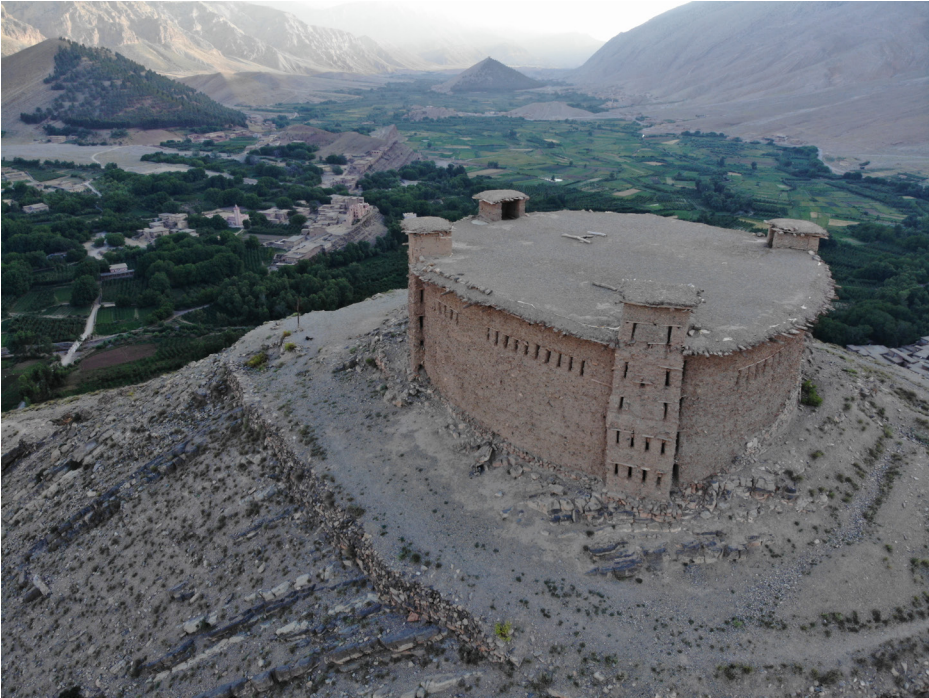
Sidi Moussa granary attic
