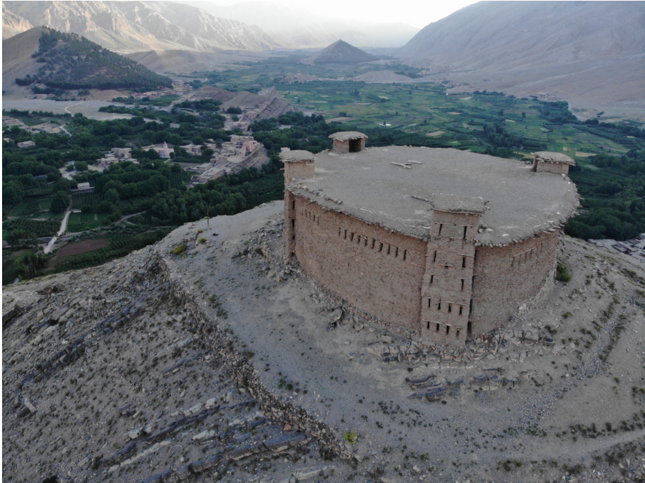
Sidi Moussa granary attic
